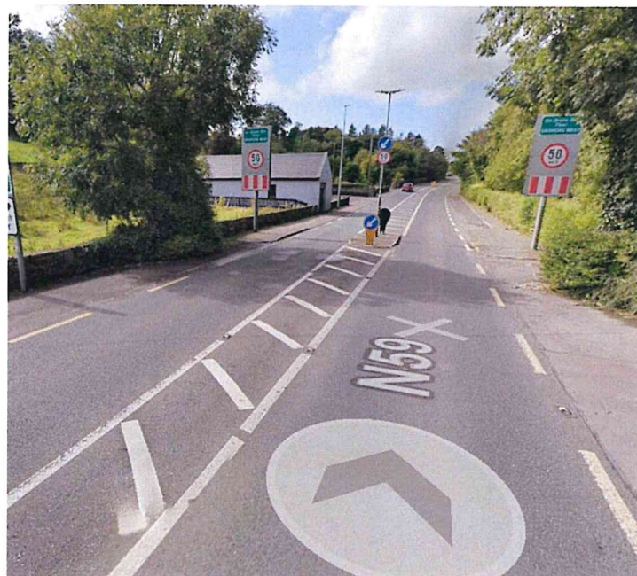
Photograph H2: The N59 entering Dromore West from the Sligo side of the village, The image shows Sean Sweeney Funeral Home on the left, also showing the 50km/h gateway signs on both sides of the road, the central traffic island with keep-left bollards, hatched road markings and street lighting. Source: Google Street View.
