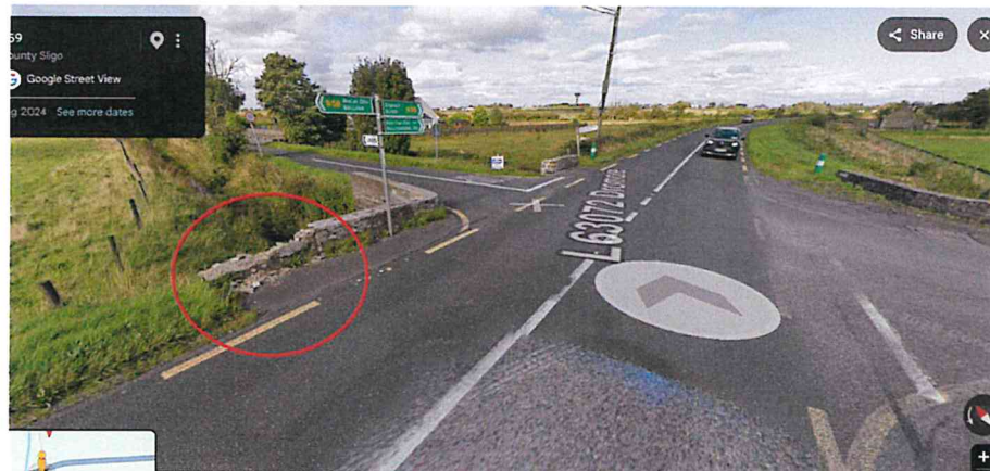
Photograph F2: The approach to Joyce's Cross on the L63072, with damage to the bridge wall circled from August 2024. Source: Google Street View.
