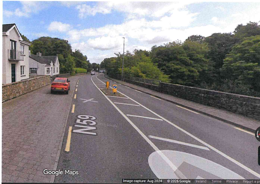
Photograph H1: The N59 approach to Sean Sweeney's Funeral Home. The view is leaving the village and heading towards Sligo. It is showing the central traffic island and bollards, street lighting and roadside parking. Source: Google Street View, August 2024.
